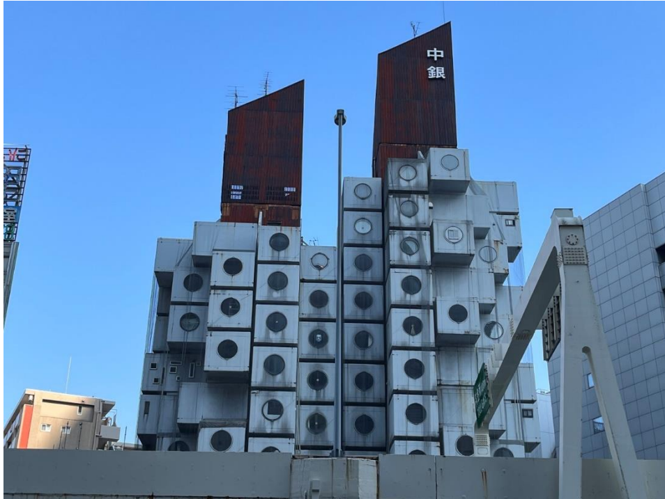
Stacked capsules with round windows visible from the highway Photo before disassembly, provided by Nakagin Capsule Tower Preservation and Restoration Project
